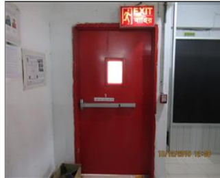
Photo of fire safety equipment Fire door.JPG
