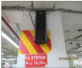
Photo of fire safety equipment Public Addressing System (PA).JPG
